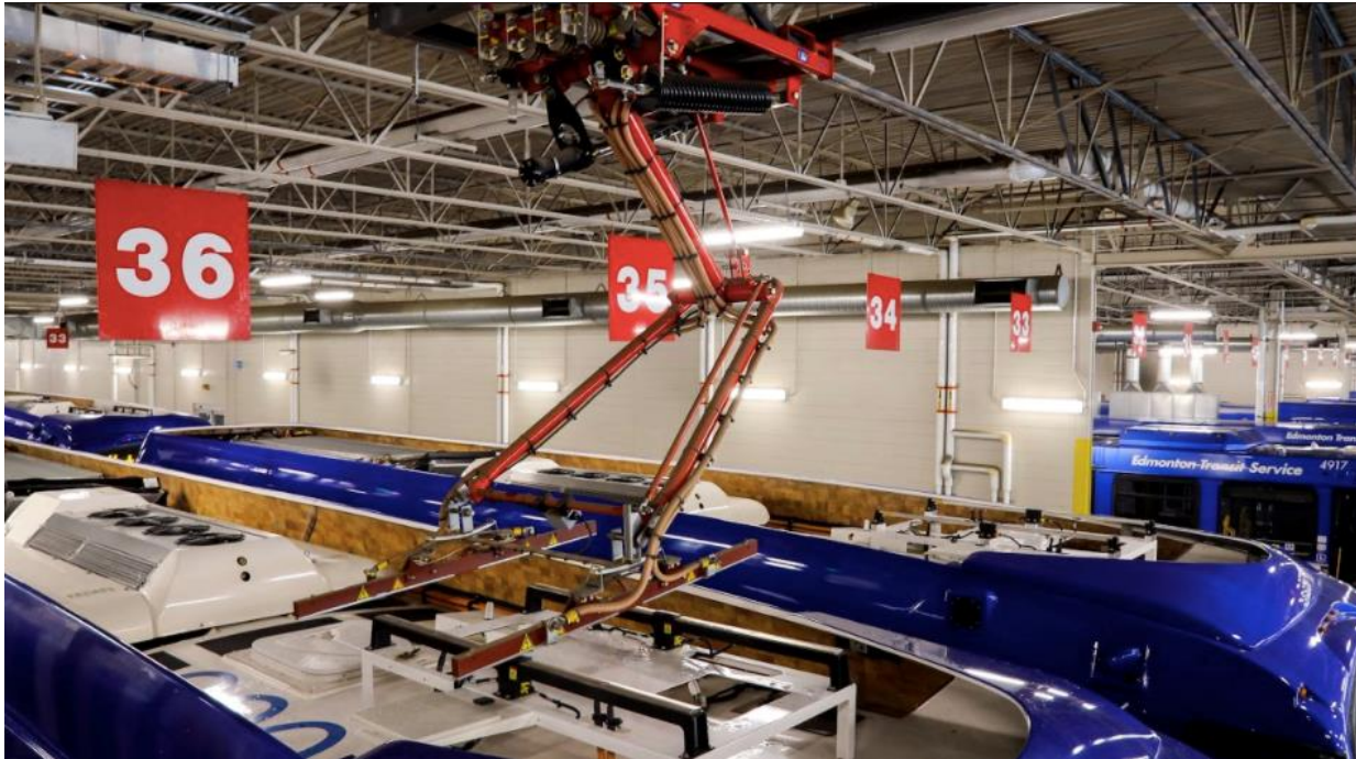
Figure 18: Overhead Pantograph Equipment for BEB Charging (Edmonton Transit, Alberta). 45
