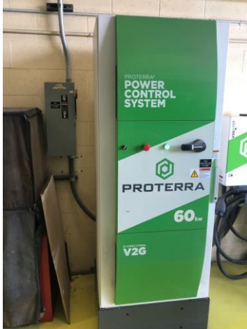
Figure 38: Charging cabinet and dispenser within maintenance bay
