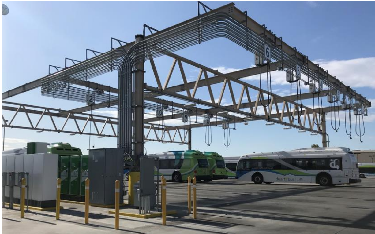
Figure 17: Clustered Vehicle Chargers (left; dotted red area) with Overhead Retractable Dispensers (Foothill Transit, California).
