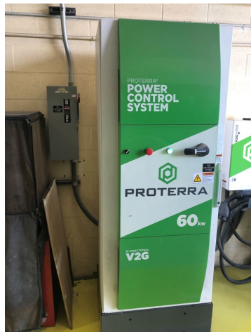
Figure 38: Charging cabinet and dispenser within maintenance bay
