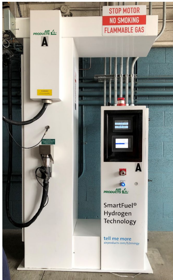
Figure 56: Hydrogen fuelling dispenser, Orange County, California.
