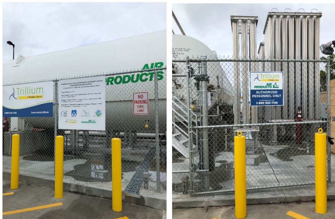
Figure 55: Liquid hydrogen storage tank and vaporizers as part of Orange County's hydrogen fuelling infrastructure.
